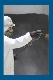
WATCHDOG H3 stays where it's sprayed to maintain consistent coverage of 40 mils cured and deliver hydrostatic head resistance up to 3 times greater than other asphalt-emulsion waterproofing products. WATCHDOG H3 is so reliable, it's backed by a 10-year transferable warranty.\*
