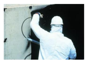
The WATCHDOG WATERPROOFING membrane is spray-applied to seamlessly bridge foundation settling cracks and seal out water penetration. Its material was specifically designed for spray application on below-grade exterior foundation walls. The membrane remains elastic at low temperatures for dependable year-round protection.
